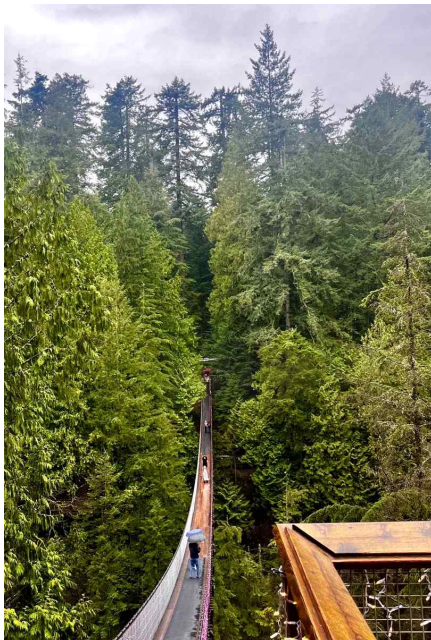
Capilano Suspension Bridge
